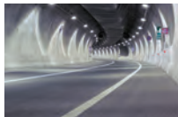
de tunnel tunnel
