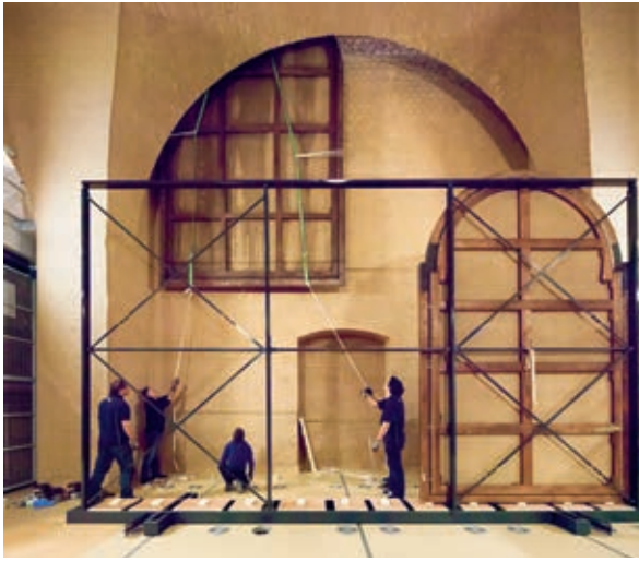
Monumental artworks are hoisted down from the Rubens Gallery to the new storage depot.
