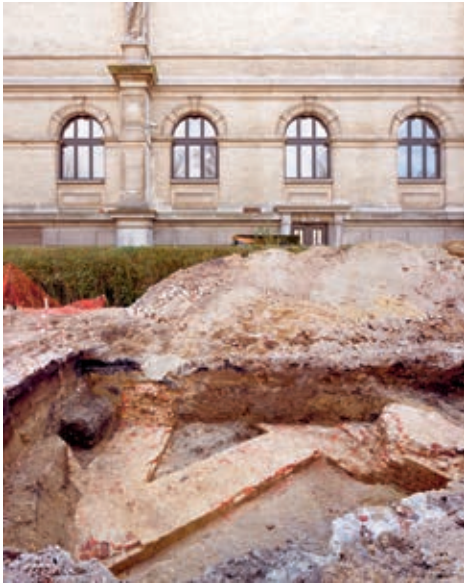
The archaeological remains of the citadel of Alva were documented during the renovation works.
