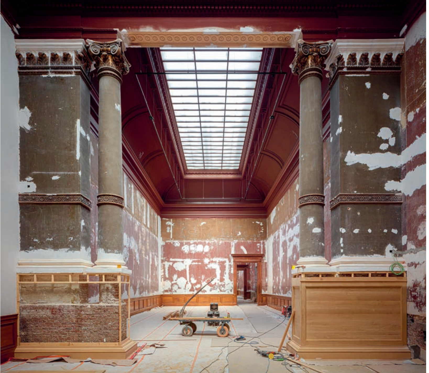
Ornamental columns were discovered behind false walls.
