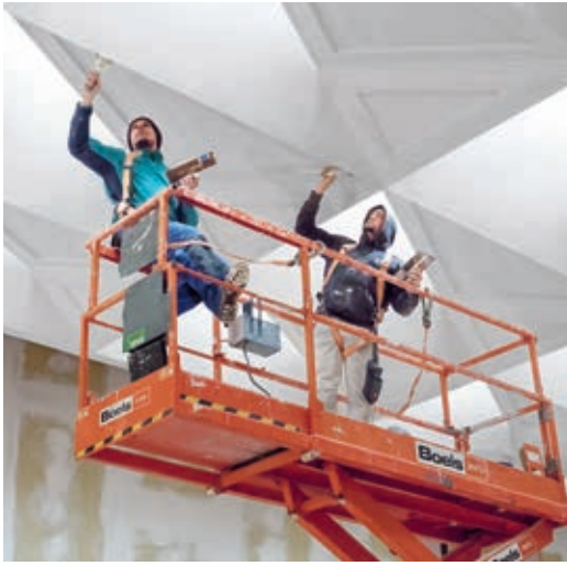
Interior finishing of the skylights.
